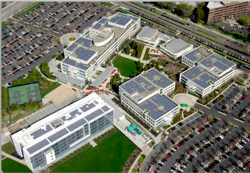
A 650-kW system on eBay headquarters in San Jose, California. (SolarCity)
